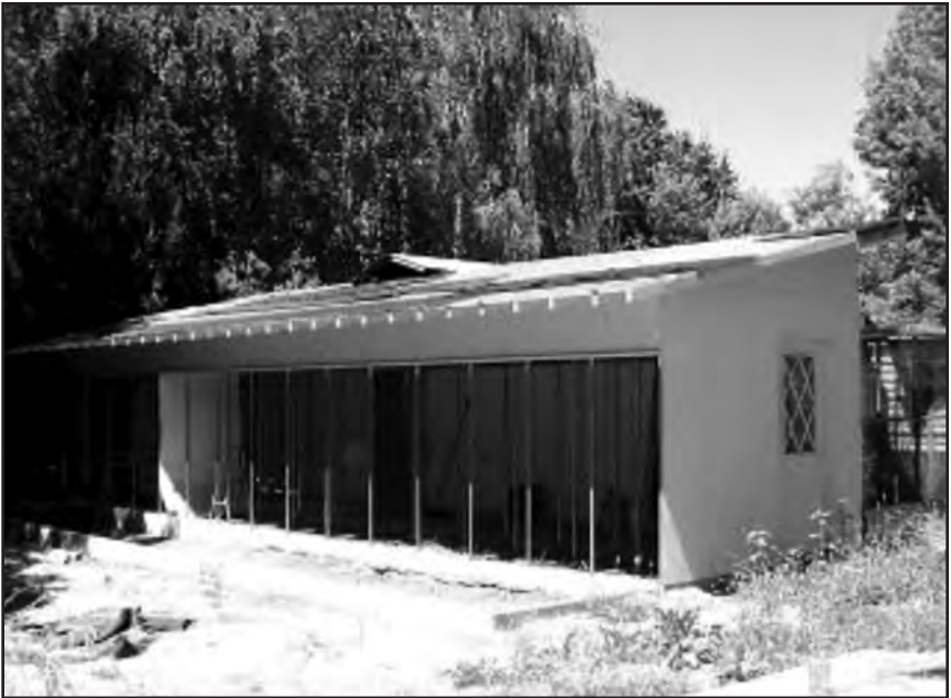
Picture taken in mid-summer showing how the overhang on the roof shades the front undercover section of the aviary so it doesn't heat up as much. In the winter, when the sun is lower in the sky, the sun shines into this area. The aviary is facing south.
