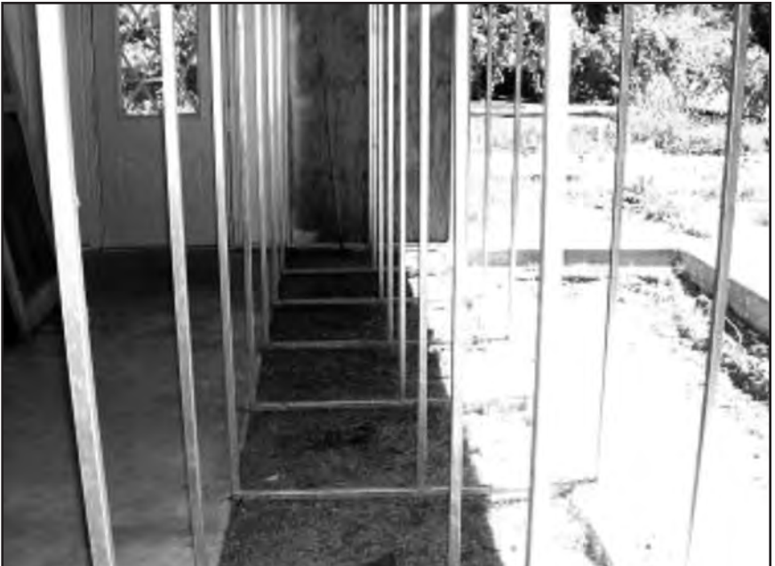
Picture showing the steel frame work that supports the structure.
