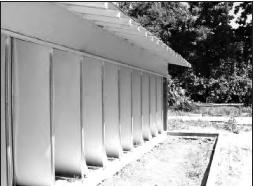
The FRP panels installed on the flight dividers.
