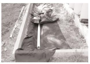
Picture showing underground drain line for outside flights. It is set in and covered with filter fabric. The fabric is used to keep the finer pieces of gravel from getting into the pipe.
