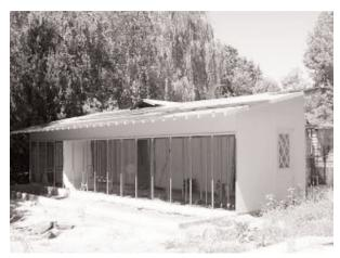
Picture taken in mid-summer showing how the overhang on the roof shades the front undercover section of he aviary so it doesn't heat up as much. In the winter, when the sun is lower in the sky, the sun shines into this area. The aviary is facing south.
