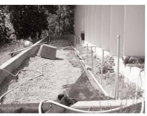
Picture showing the water main line with the services coming up at each flight. This area gets covered with gravel to within 2 of the top of the foundations.
