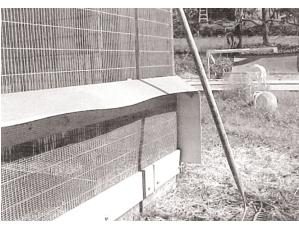
Picture showing ½" X ½" wire with flashing so rats or mice can't climb to the top of the aviary.
