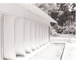
The FRP panels installed on the flight dividers.
